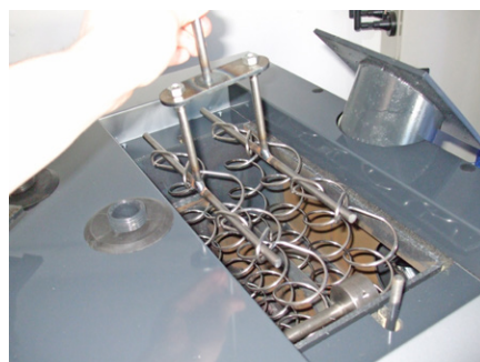
6. Remove the Turbulator lift and the Turbulator springs.
