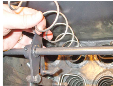
6. Replace the Turbulator springs.
