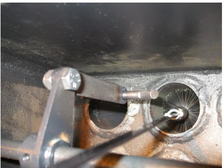
5. Sweep the convection pipe surface with a brush. Remove any ash. Make sure to insert the brush all the way down the convection pipes. Repeat a couple of times.
