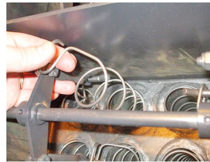
3. Remove the Turbulator springs.
