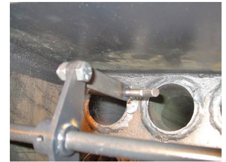
4. Turbulator springs removed.
